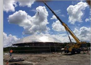
**EVERSTORE® DOMES by UIG** are built using a triangulated profile system, covered with triangular panels.
